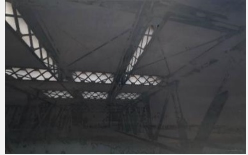
QUEEN STREET BRIDGE
